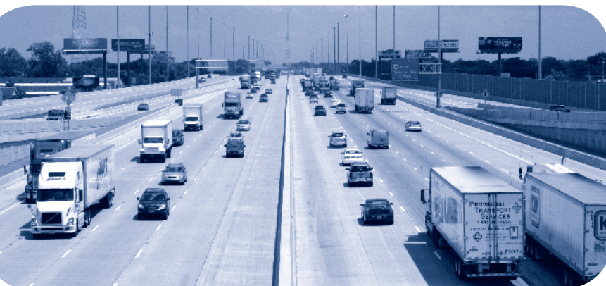
Photo courtesy of the Illinois Department of Transportation.
