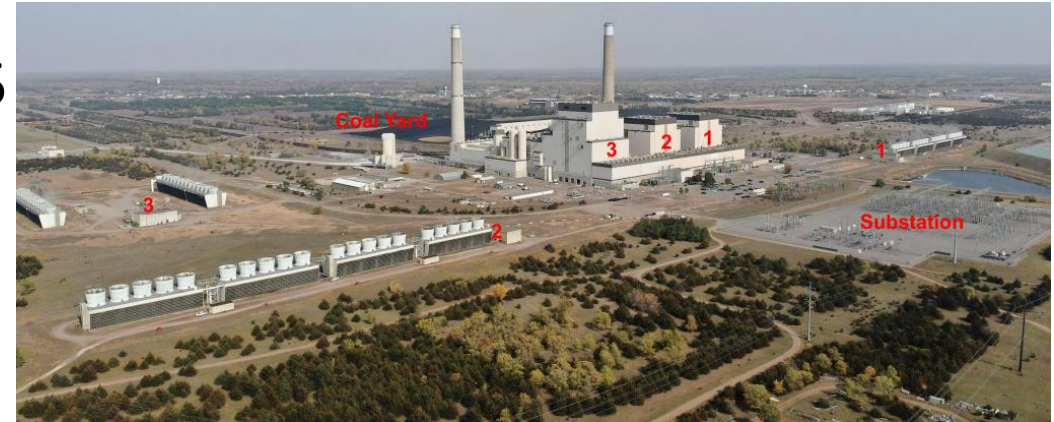
Becker, MN Power plant. Unit 2 closing this year
